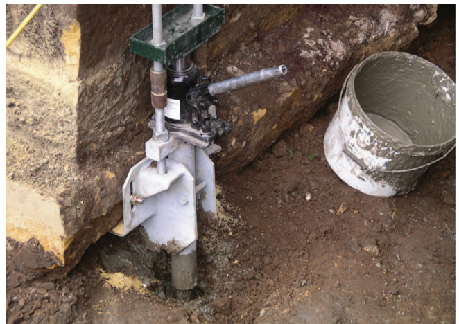
FIGURE 7. FOUNDATION BRACKET AND LEVELING JACK USED AT FOREST LODGE.
