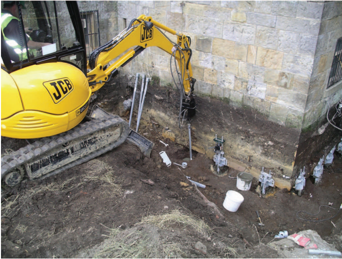
FIGURE 9. INSTALLING SCREW-PILES AT FOREST LODGE.
