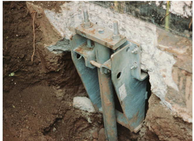
FIGURE 6. HEAVY DUTY FOUNDATION BRACKET ATTACHED TO EXISTING FOUNDATION.
